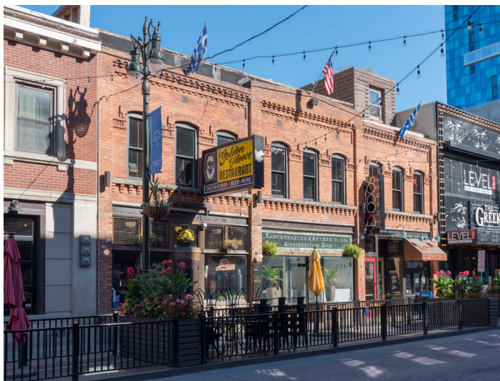
Most of Greektown's low- and mid-rise development, dating back to the 19th and early 20th centuries, is built of red brick.
