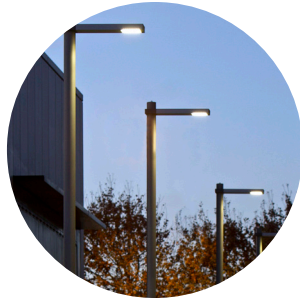
Street Lighting (20' H)
