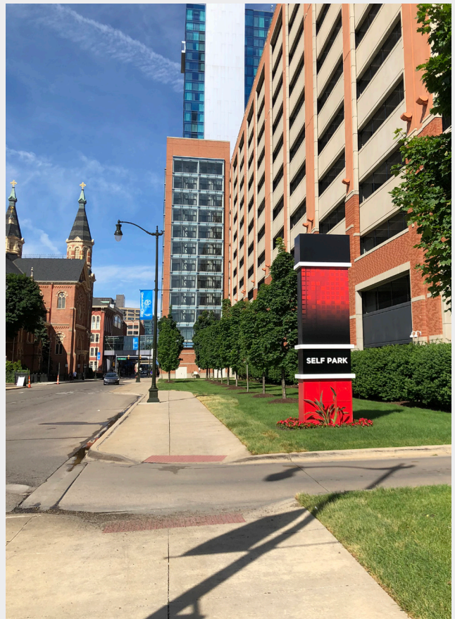
The wide frontage area is largely unusable today. Future development lining the garage should not impact garage entries and exits on Monroe Street.
